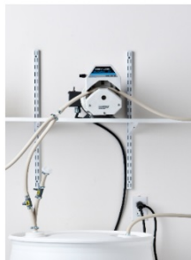
Step #8 - Start Pump and let run for 15 minutes to mix contents
